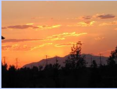
Transmission lines carry power over extended distances along Utah's Wasatch Front.
